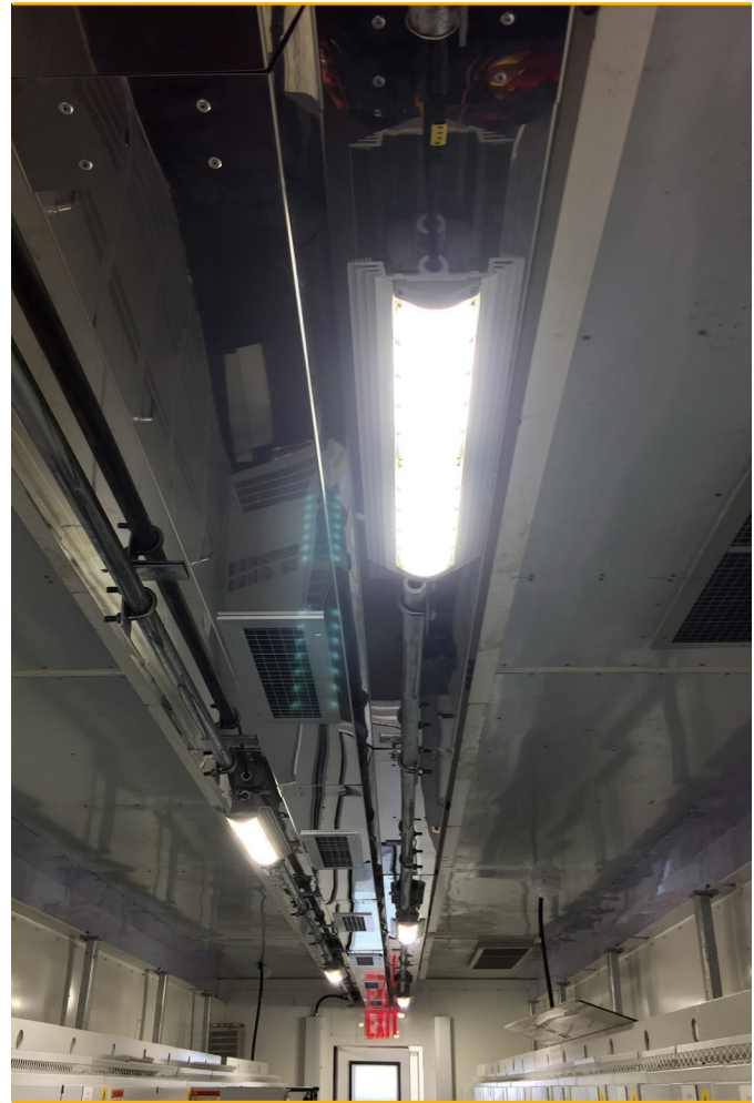
HDL2s in an electrical control room
