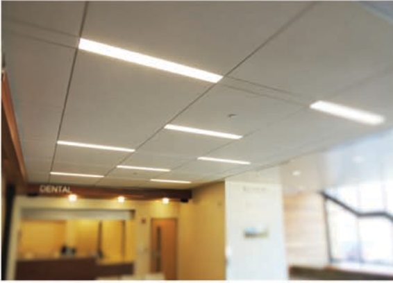
Flush with 15/16" grid (T1W)
