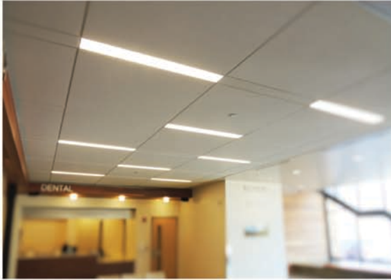
Flush with 15/16" grid (T1W)
