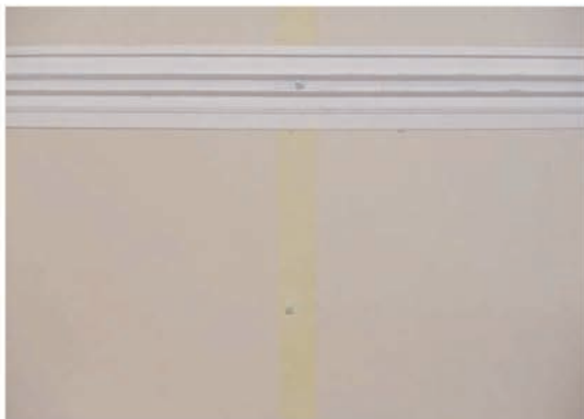
1) Plaster Rail is affixed to wall at a predetermined location prior to finishing.
