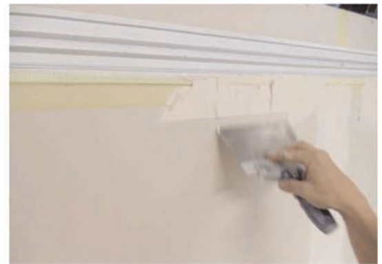
2) Plaster or other compound is blended over the lower portion of the Rail and feathered down the wall, eliminating minor inconsistencies in wall straightness.
