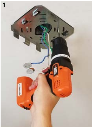
Mount plate to junction box.
