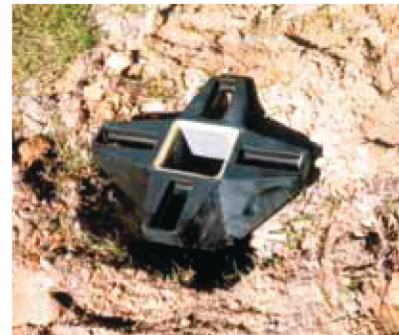
2 Backfill and tamp and pull wiring.
