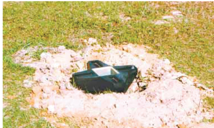
2 Backfill and tamp and pull wiring.
